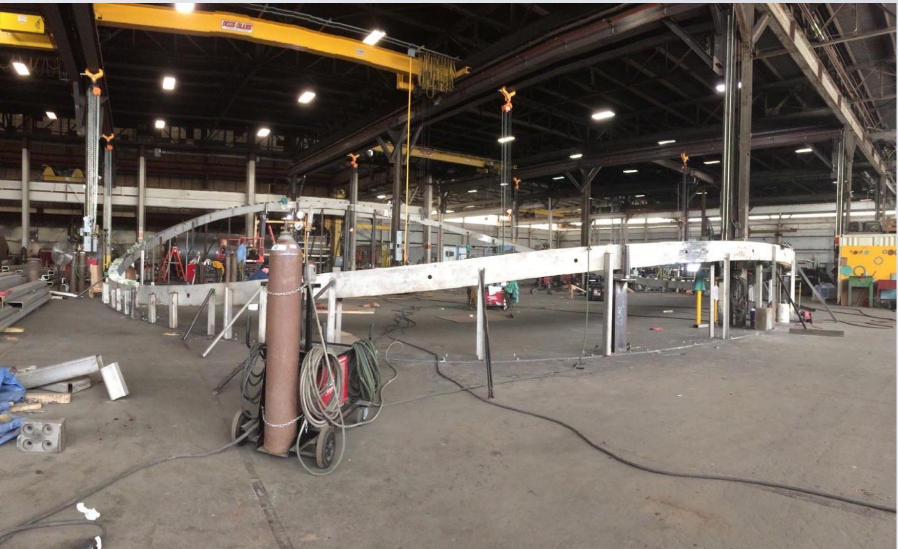
Making the giant Ring Girder
